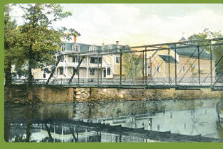
Hotel Bridge, 1880 Pratt Iron Through Truss, Leeds
